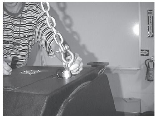
Hang the SB-1 so that the weight of the speaker is supported by the rigging hardware.
